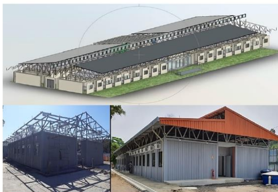
Figure 1. Isometric and panoramic construction view.
