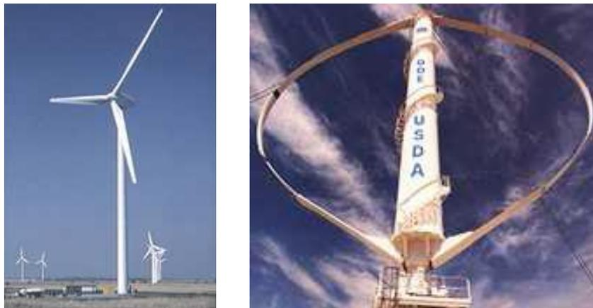
Figura 2-2. Turbina de eixo: (a) horizontal, CRESESB (2013) (b) vertical, SANDIA (apud CRESESB, 2013)
