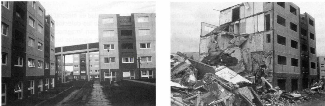
Figura 31 – School Street Hebburn – 900 casas demolidas (1987 – 1989)
